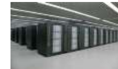
Tianhe-2 supercomputer in China
