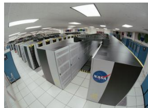
NASA Advanced Supercomputing (NAS) Facility
